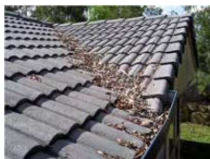
Figure 5. Image of flammable debris on a roof that could ignite from wind-blown embers, reflecting how vegetation near or overhanging structures could increase the likelihood of structure loss.
