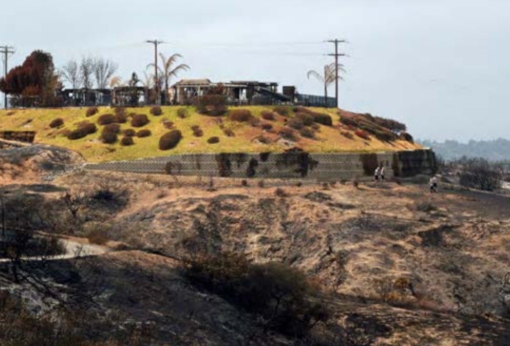
Most homes don't burn from direct contact with flame. Here, a wind-driven fire carried embers over cement and ice plant to the house, reinforcing the importance of reducing the flammability of the home—focusing fire risk reduction from the “house outward.” [Photograph by Rick Halsey]
